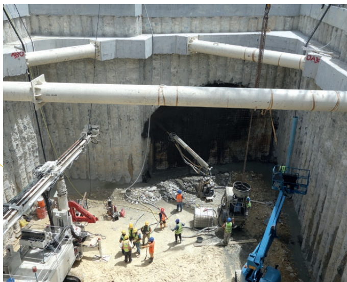
INFRASTRUCTURES (TUNNELS, OUVRAGES D'ART)
