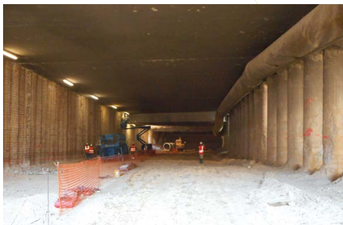
INFRASTRUCTURES (TUNNELS, OUVRAGES D'ART)
